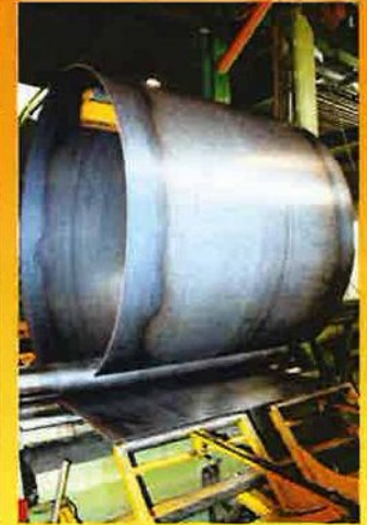
Tank rolling in progress
